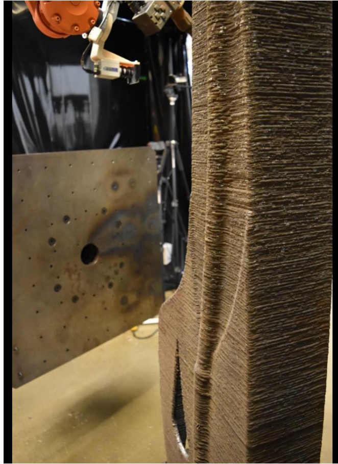
Figure 42. Support plate and hydraulic line close up.
